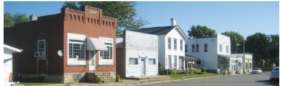
North side of Vinton Street in Old Palo
